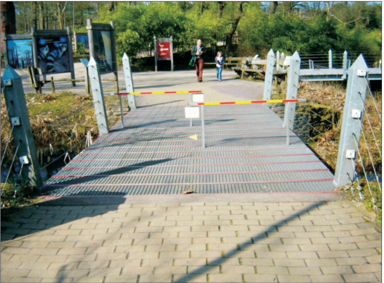
Fig.72. Use of electrical barrier-walk-through.
