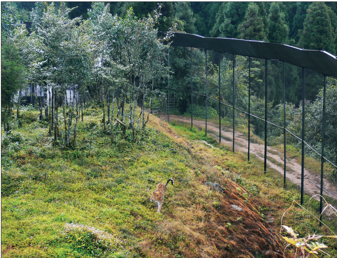
Fig.15. Open top enclosure using overhang with inclined inward and welded steel plate on chainlink mesh fence as a barrier for leopards at Himalayan Zoological Park, Gangtok.
